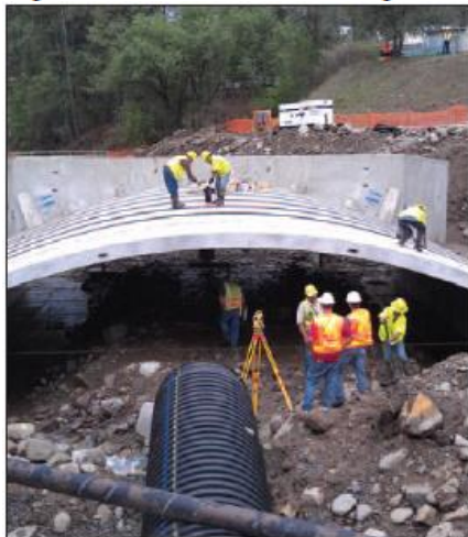
Zia Engineering conducts a construction inspection for the Eagle Bridge project.
