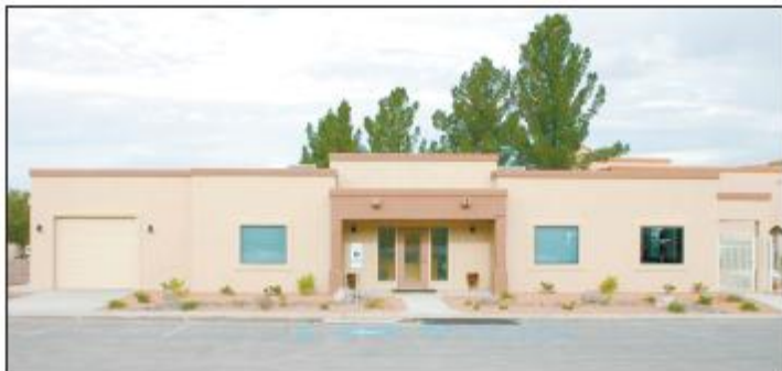
Sharon Wasser of Organ Vista Builders recently constructed this office building for the Pinnacle Management Group in Las Cruces.
