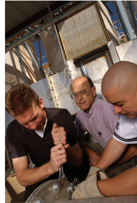
NMSU engineering technology students Jeff Nelson of Albuquerque, left, and Roberto Briones of Las Cruces, right, tighten a bolt on a filter test facility designed and built as a senior class project. Faculty member Craig Ricketts looks on.
